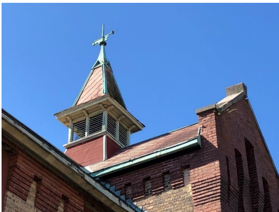
Detail showing brick corbelling at roofline and belfry.
