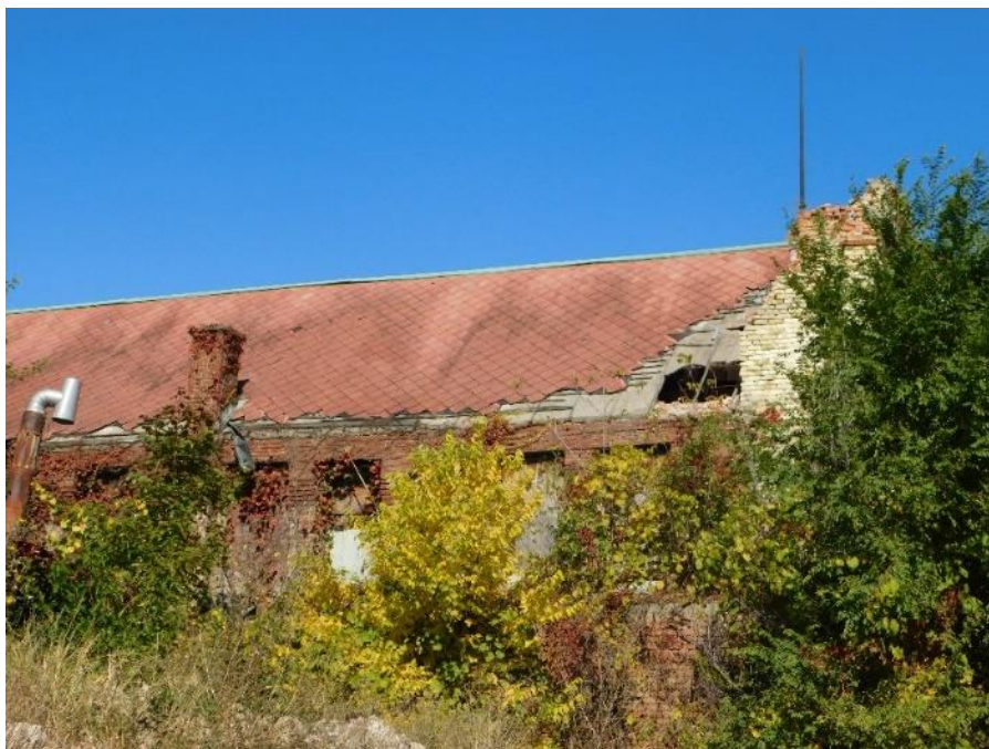
View of deteriorated roof with a gaping hole in it, looking northwest.
