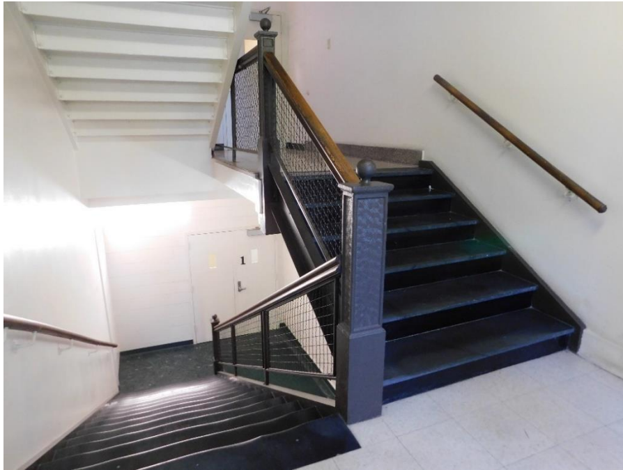
View of the only stairway in the 1914 Dormitory to retain its original iron newell posts and railings following a gut renovation that took place in the mid-1980s.
