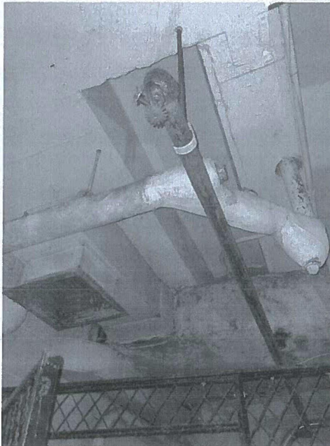
Visible suspect Asbestos-Containing Materials: Aircell and Mud, Thermal Insulation on Pipes and Ducting throughout.
